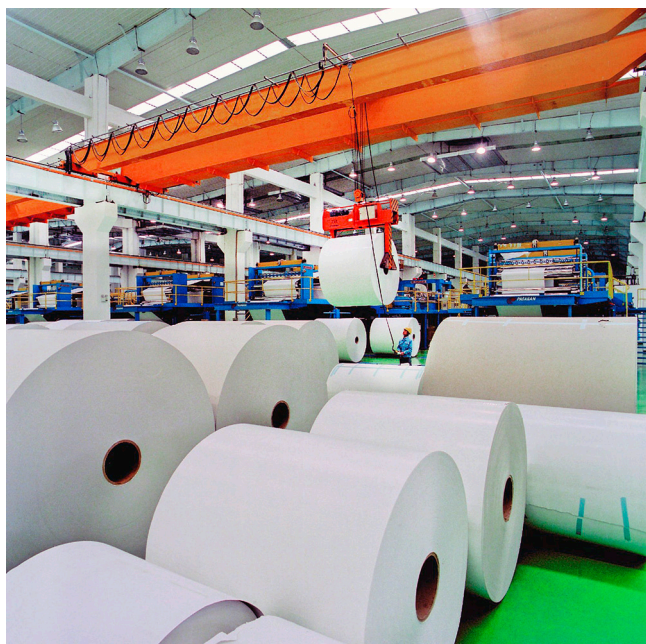
Industry crane system
