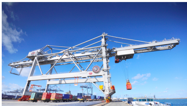
Harbor crane system
