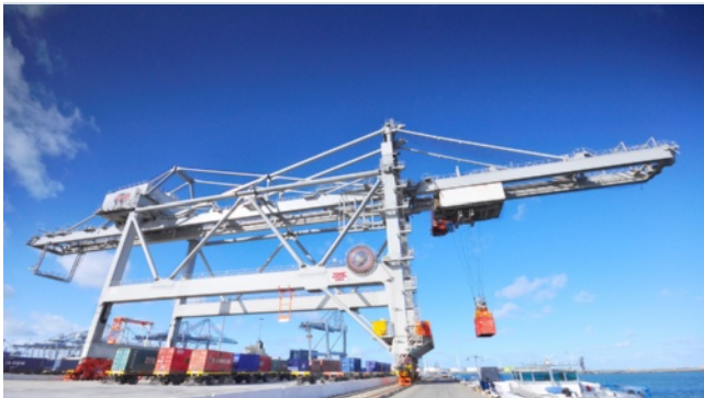
Harbor crane system
